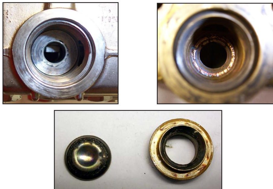
Figure 5-2. Inspect Manifold and Old Valves
